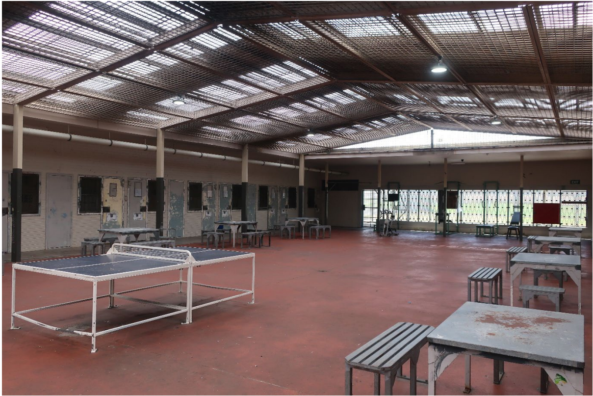
Photo 1: The internal courtyard of Unit 1 A Yard.
