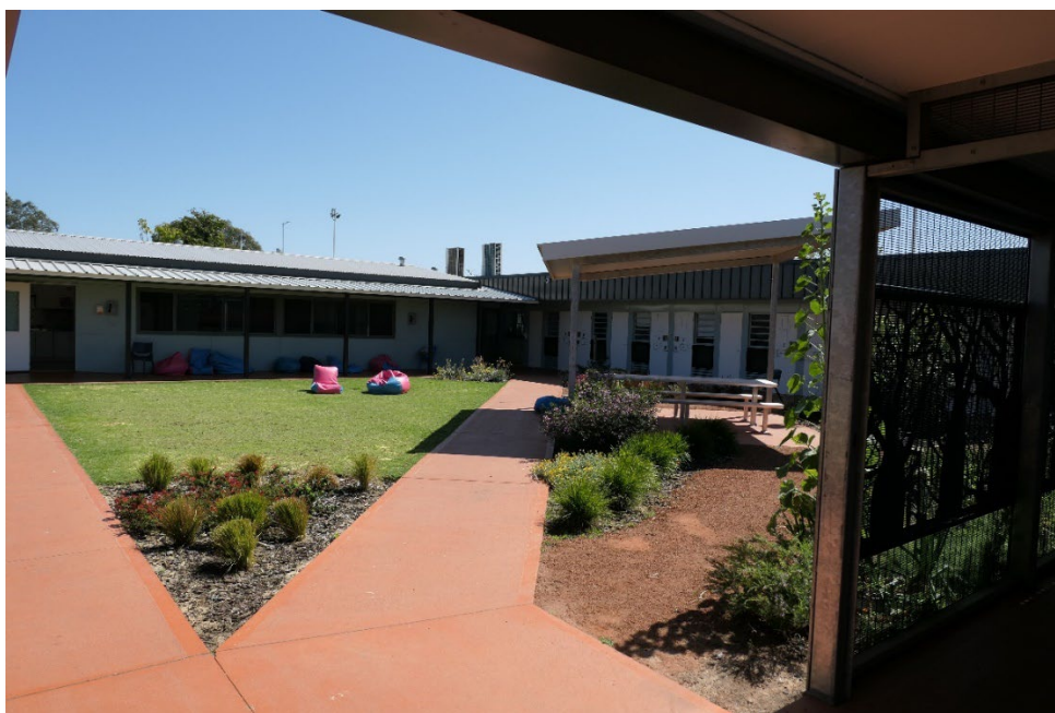
Photo 1: Bindi Bindi Unit shared internal open yard.
