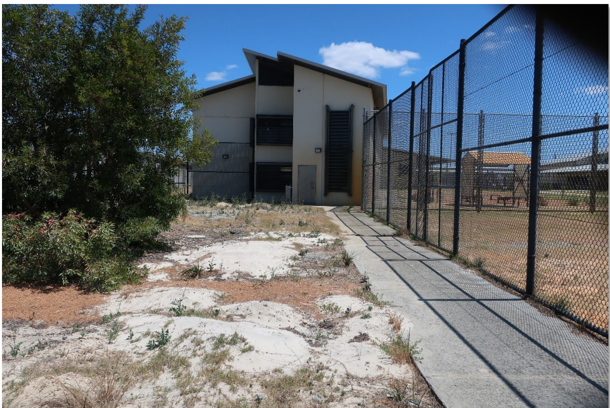
Photo 4: The yard attached to the management cells was currently unused.
