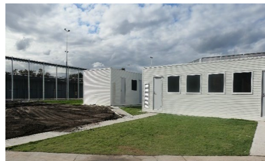
Photo 5 Transportable buildings installed in the Jasper precinct meant to reduce movement of young people from the unit.
