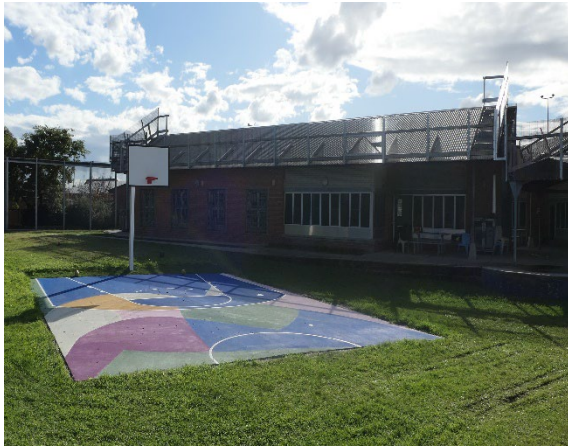
Photos 3 and 4 Anti-climb roof treatments installed as part of target hardening approaches at Banksia Hill.
