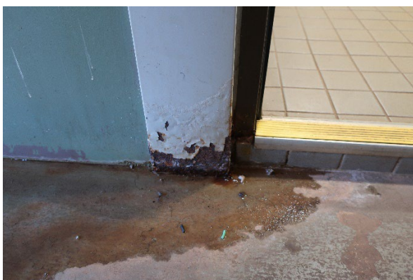
Photo 4: Structural corrosion
