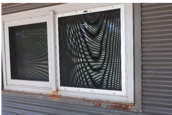
Photo 6: External corrosion
