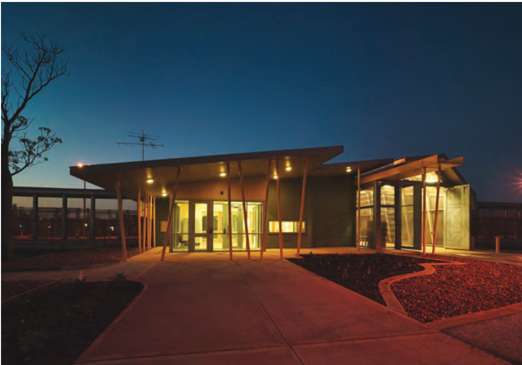
Photo 3 : West Kimberley Regional Prison entrance.
