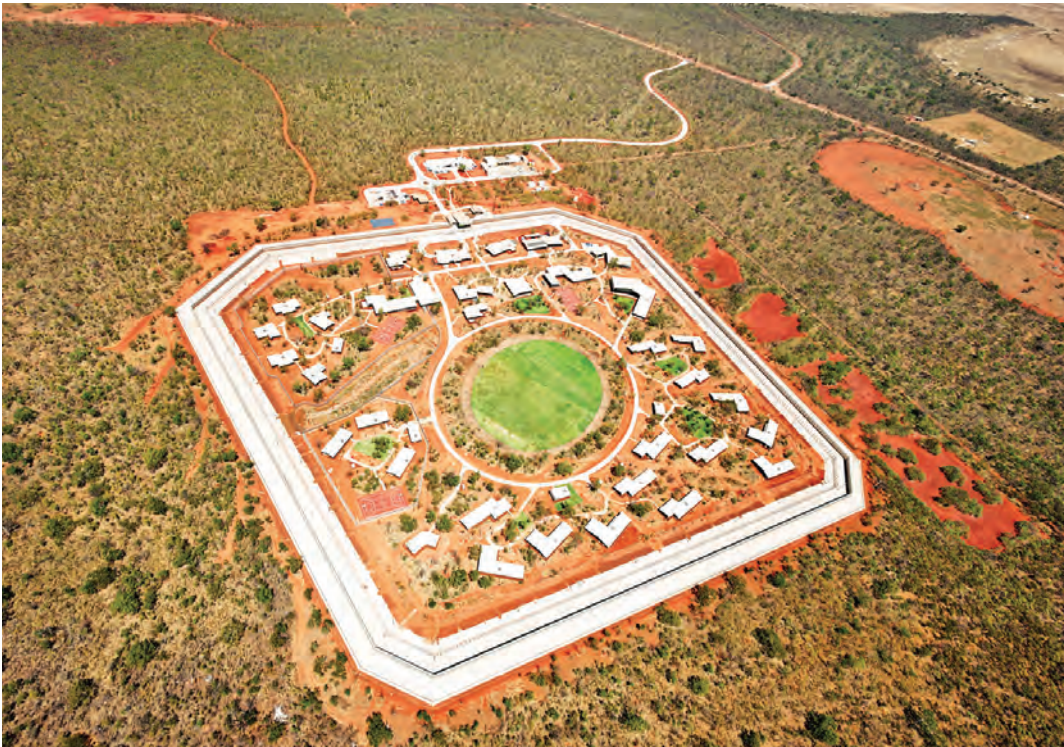
Photo 2 : Aerial photo of West Kimberley Regional Prison.
